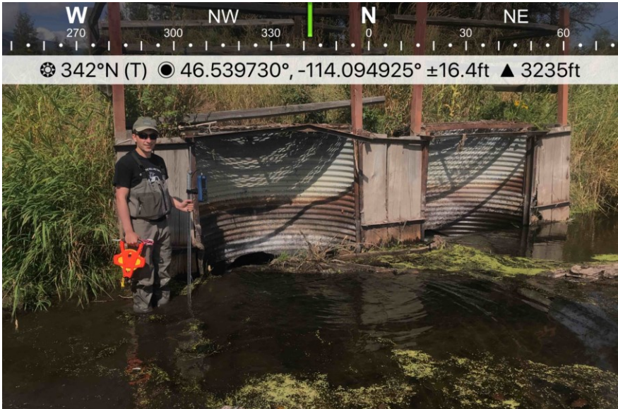
This relic water control structure near the mouth of North Burnt Fork Creek, prevents fish passage and obstructs natural sediment and flow processes. This barrier will be removed and replaced with a pedestrian bridge.
