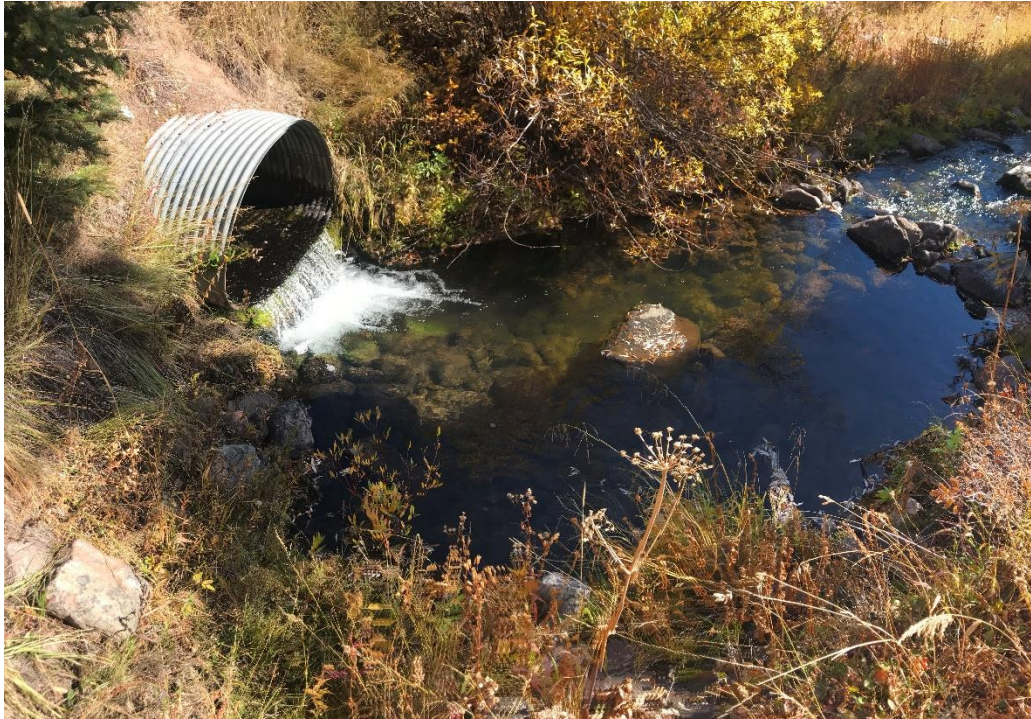
Figure 20. Perched culvert at FS RD 6406 crossing on Coyote Creek (46.8650, -110.8398).
