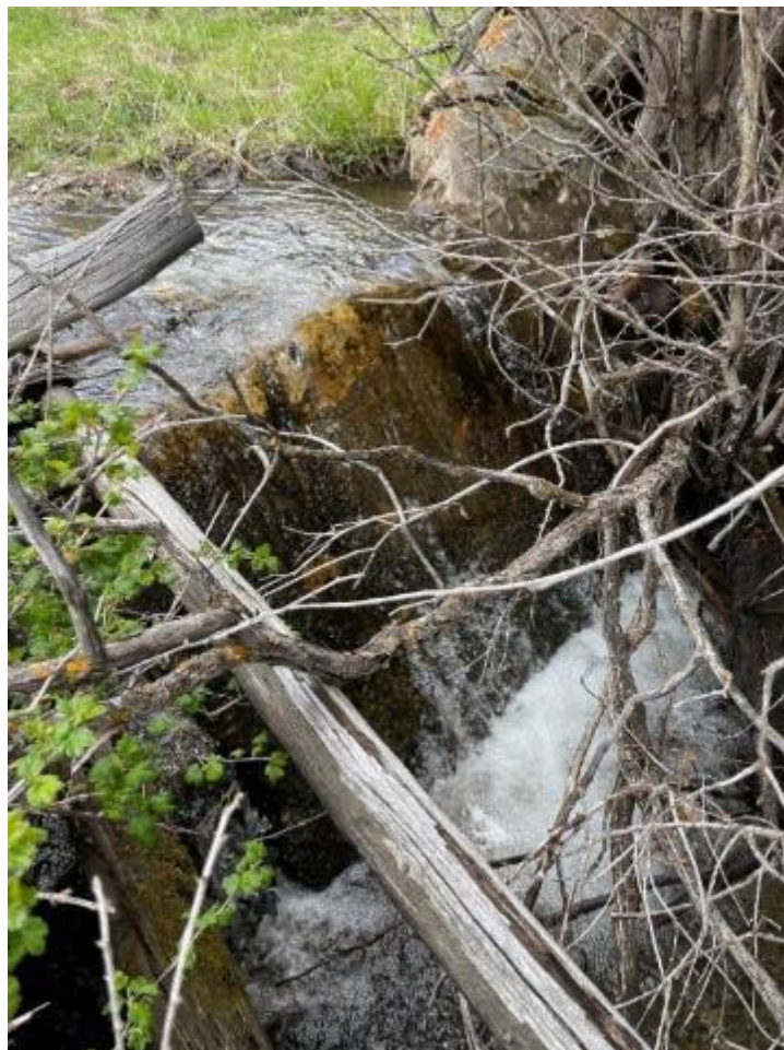
Figure 32. Concrete slab in Pickfoot Creek located at 46.57756, -111.24741.
