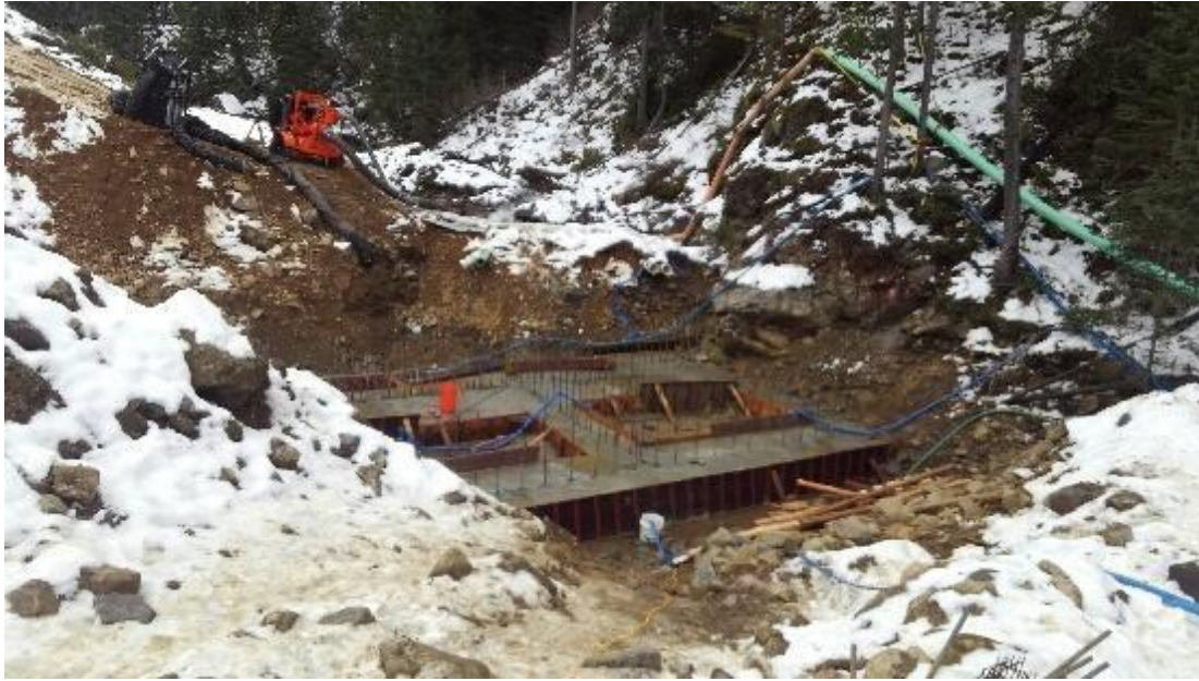
Figure 4. Concrete footer at Carpenter Creek fish barrier construction site.
