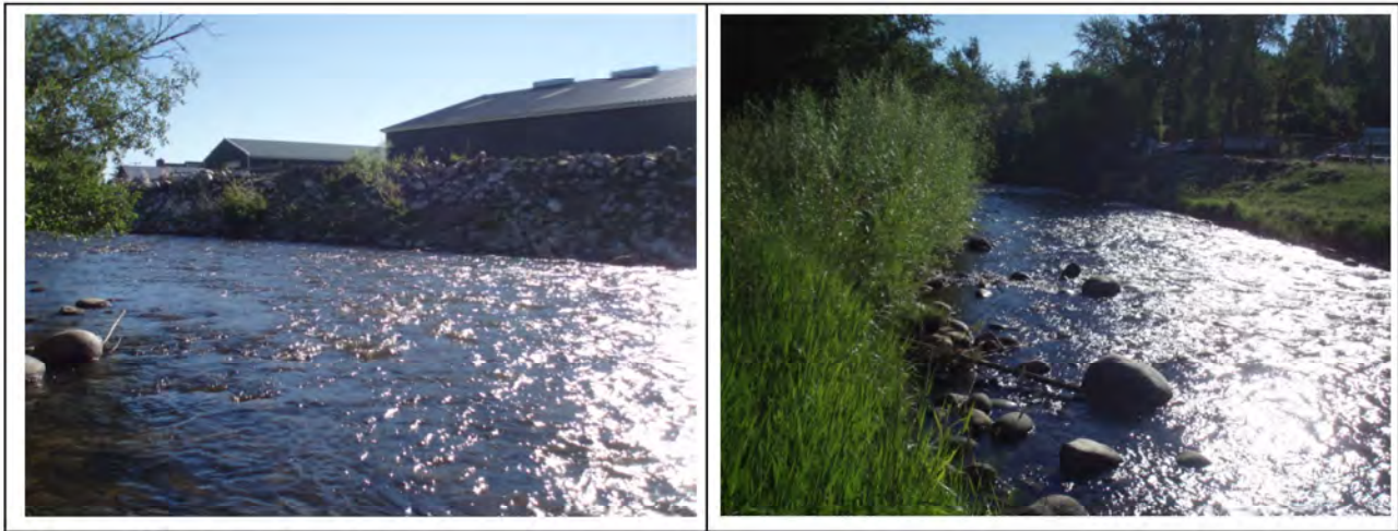
Armored bank on river right to protect property at F30.
