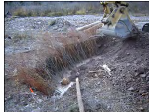
EXAMPLE OF A WILLOW TRENCH INSTALLATION
