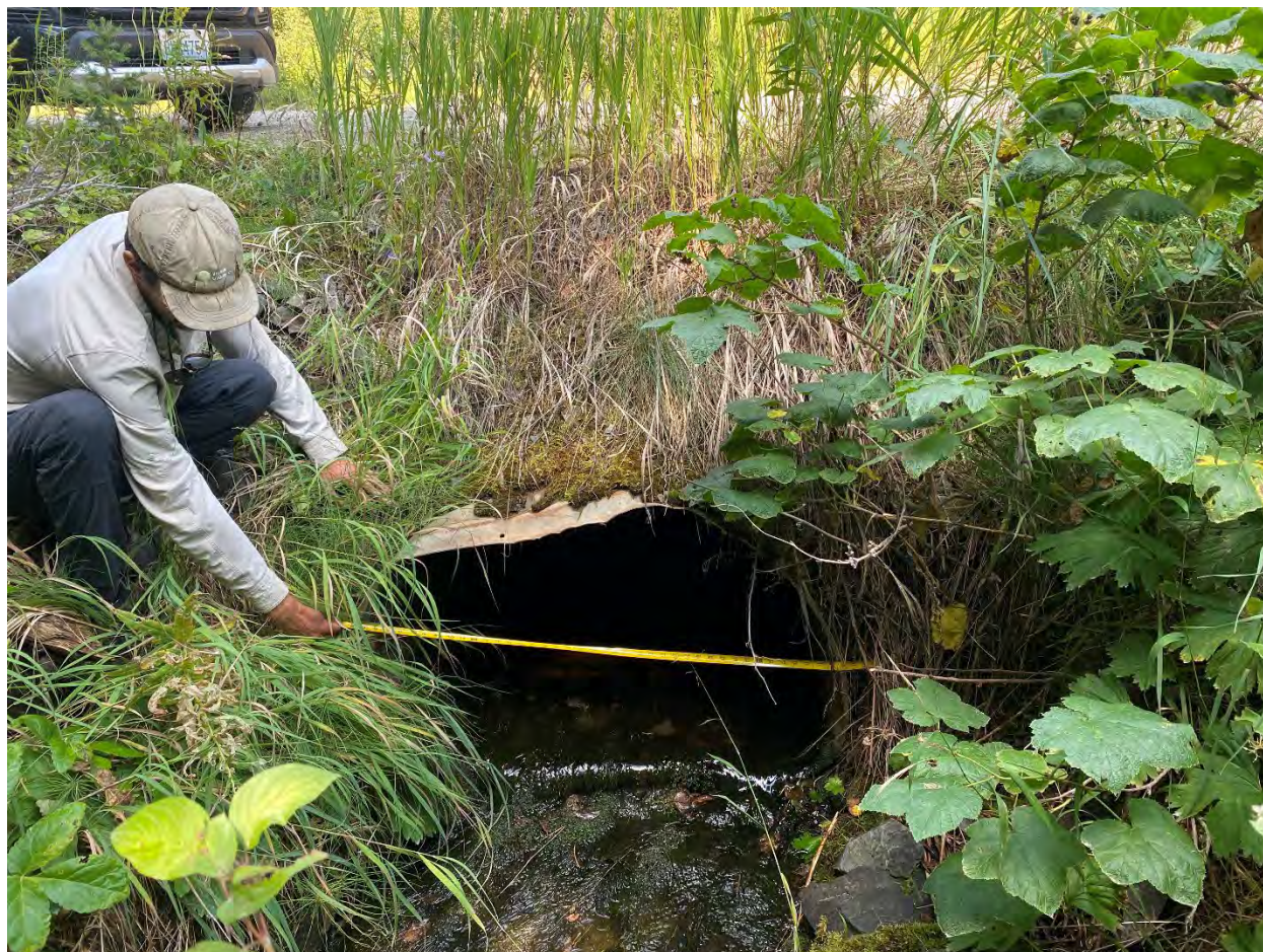
Figure 1: 42 inch x 24 inch culvert outlet.
