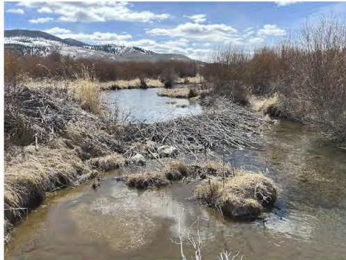
BEAVER DAM LOOKING UPSTREAM (SOUTHWEST), STA 25+00
