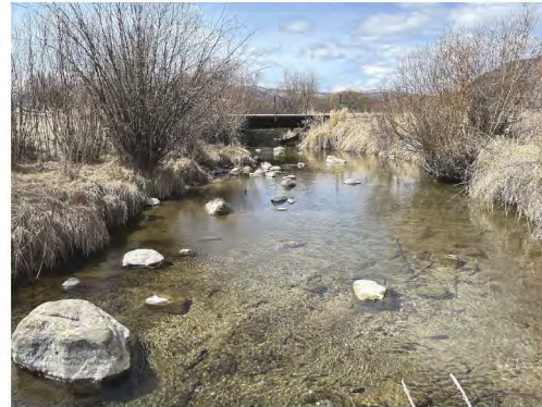
BRIDGE NEAR CONFLUENCE LOOKING UPSTREAM (SOUTHWEST), STA 2+00
