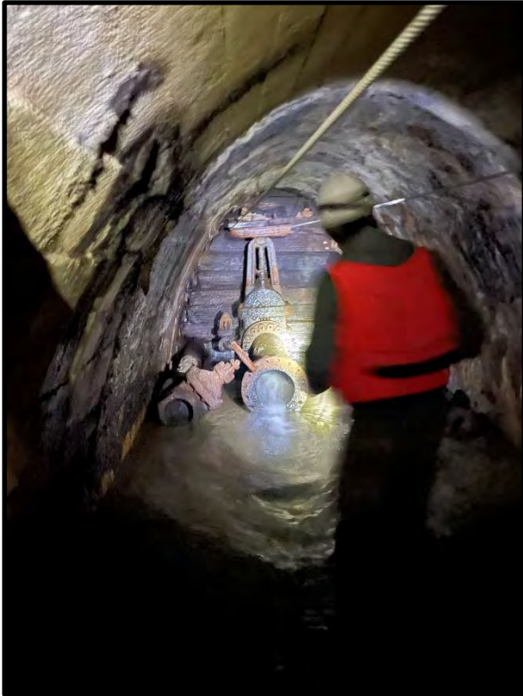
Outlet Conduit near bulkhead showing cable and wheel on top of valve operator. Valve operator broken connections ( 5 of 6 are broken).
