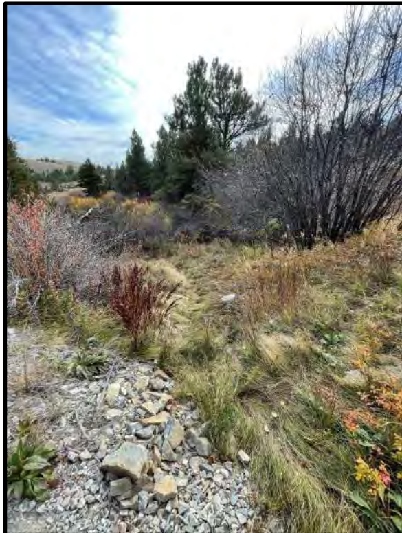
Vegetation on downstream face
