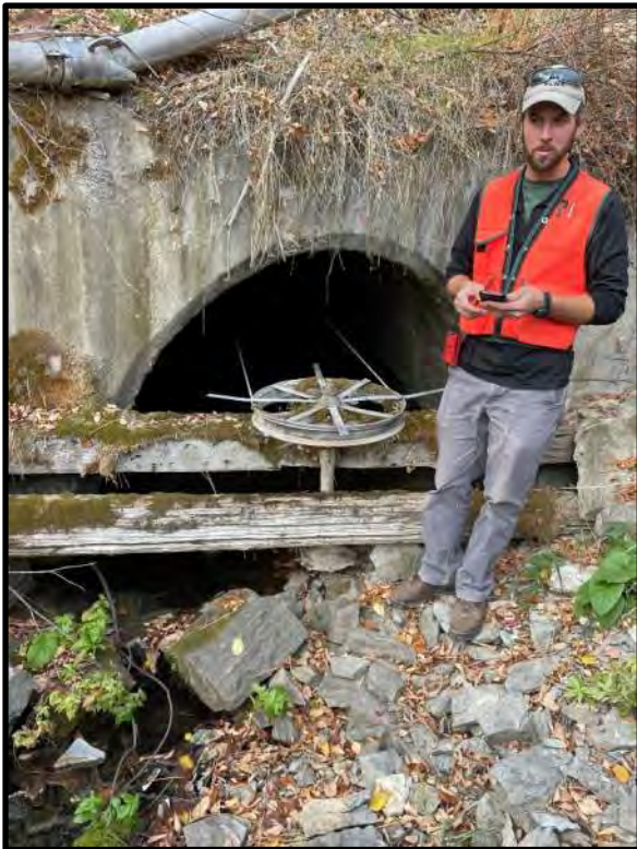
Conduit entrance, outlet pipe pulley and cable
