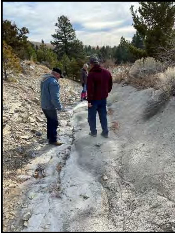
Primary spillway channel; concrete patching on right side
