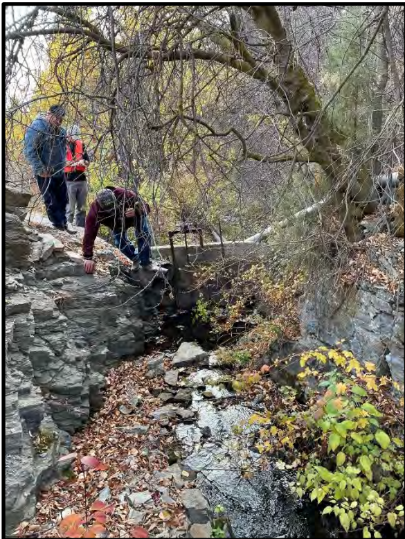
Outlet channel and irrigation headgate
