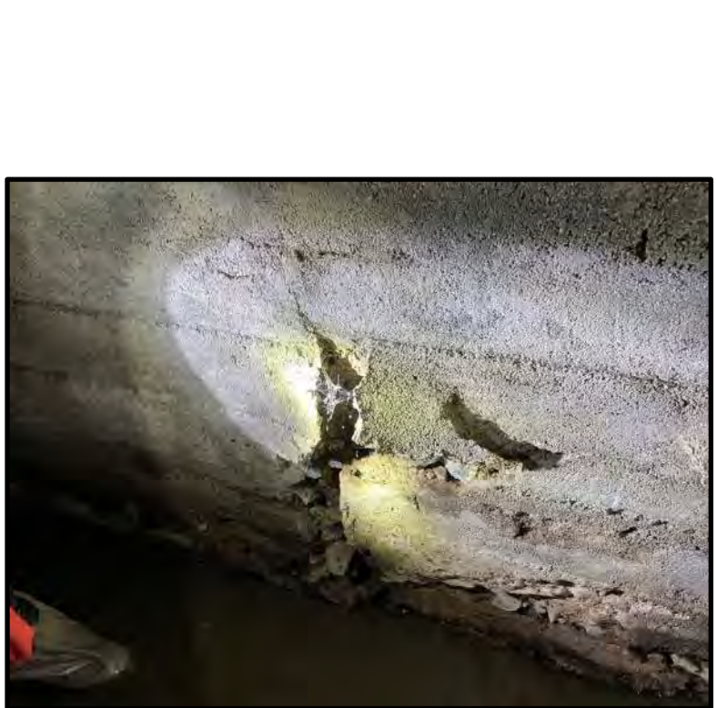
Concrete spalling on conduit wall
