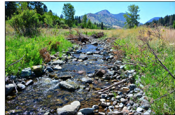
TYPICAL CONSTRUCTED STREAMBED THROUGH A RIFFLE FEATURE
