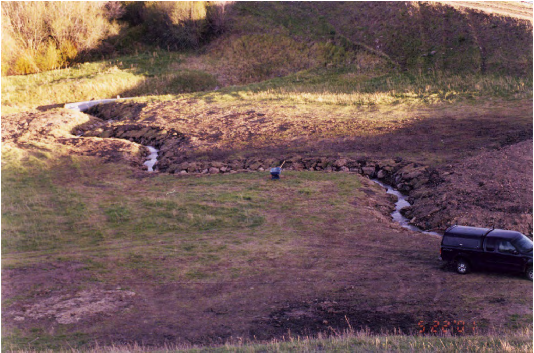
Figure 4. Bypass channel looking downstream to the dam outlet pipe, 2011.
