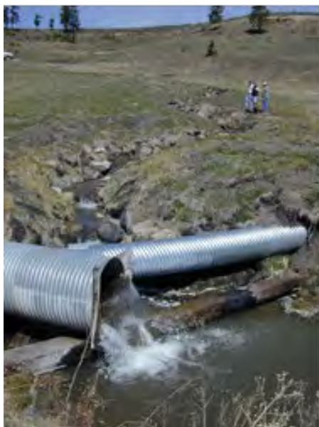
Figure 2. Existing bypass channel looking upstream from the dam outlet in the early-2000s while the channel was still functional.
