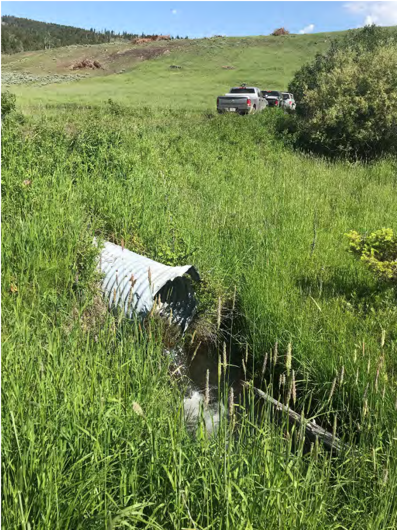
Figure 5. Overflow channel at the upper reservoir and existing culvert at the dam road crossing, 2022.
