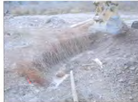
EXAMPLE OF A WILLOW TRENCH INSTALLATION
