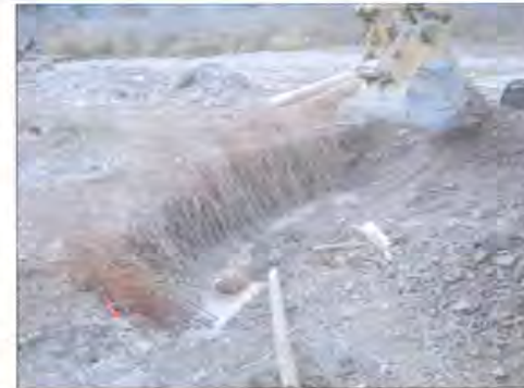
EXAMPLE OF A WILLOW TRENCH INSTALLATION
