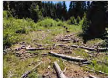
EXAMPLE OF CONSTRUCTED FLOODPLAIN ROUGHNESS
