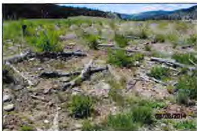
EXAMPLE OF CONSTRUCTED FLOODPLAIN ROUGHNESS
