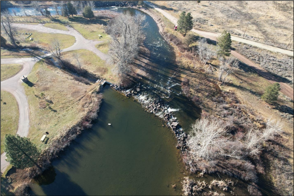
Photo 3. Oblique view of Clearwater River diversion dam and project reach.
