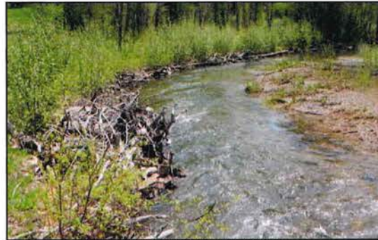
TYPICAL CONSTRUCTED STREAMBED THROUGH A RUN FEATURE
