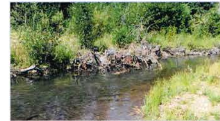
EXAMPLE OF A LARGE WOOD STRUCTURE
