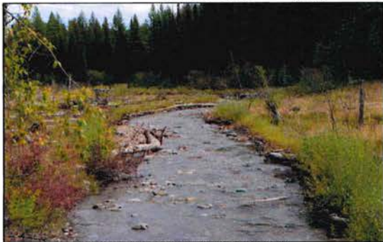
TYPICAL CONSTRUCTED STREAMBED THROUGH A RIFFLE FEATURE
