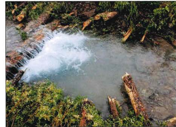
EXAMPLE OF A CONSTRUCTED LOG STEP POOL
