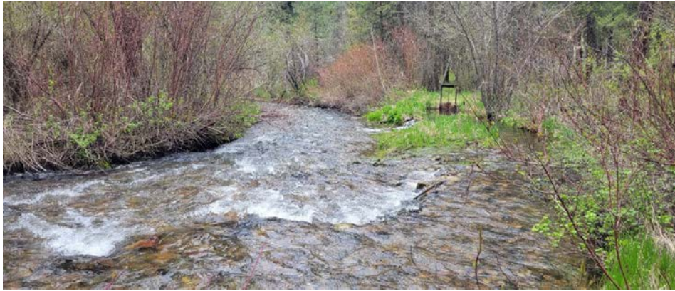
Figure 2. Looking downstream at the Gratton Diversion and headgate on the right side of the channel. Photo taken June 2022. GPS Coordinates: 46.5759, -113.6639
