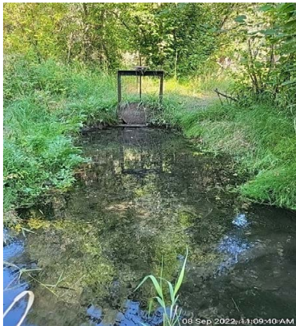
Figure 4. Headgate for the Gratton Irrigation Diversion ditch. Photo taken September 2022.
