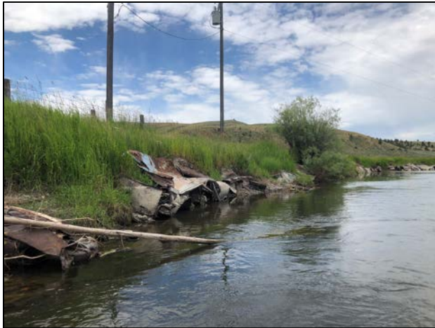
Figure 78. Car bodies used as bank stabilization along the Smith River upstream of Camp Baker.
