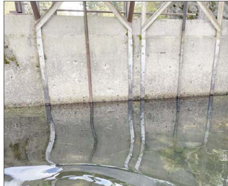
VIEW OF EXISTING HEADGATE FRAMES (4/18/2022)
