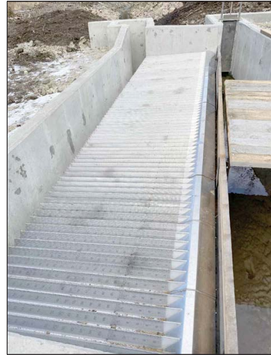
VIEW OF CORRUGATED WATER SCREEN PANELS
