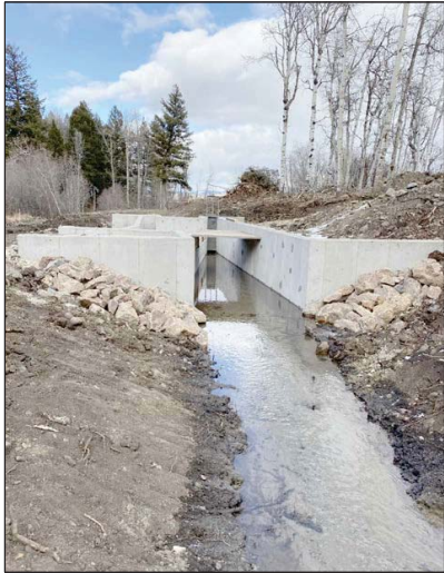
VIEW OF UPSTREAM END OF FISH SCREEN STRUCTURE
