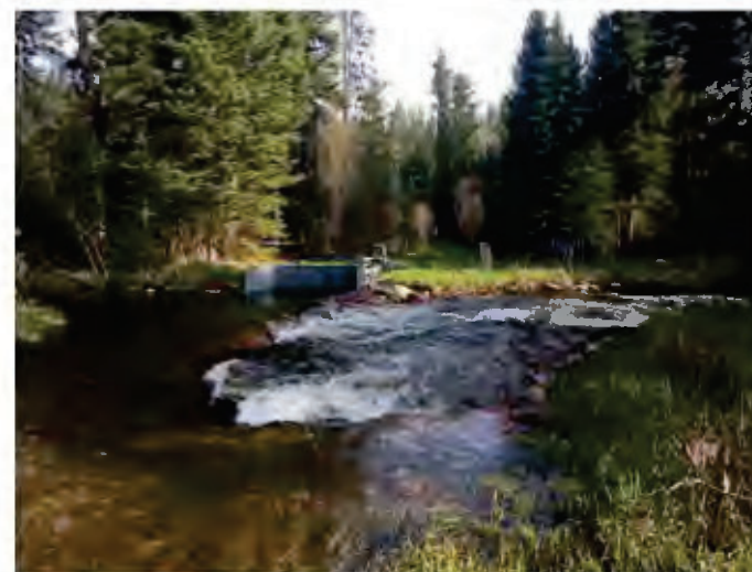
EXAMPLE OF A SIMILAR BOULDER CASCADE STRUCTURE WITH DIVERSION
