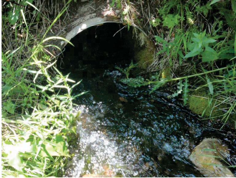
Inlet and outlet of the upper noname creek culvert. It will be replaced with a 60-inch hydraulic culvert.
