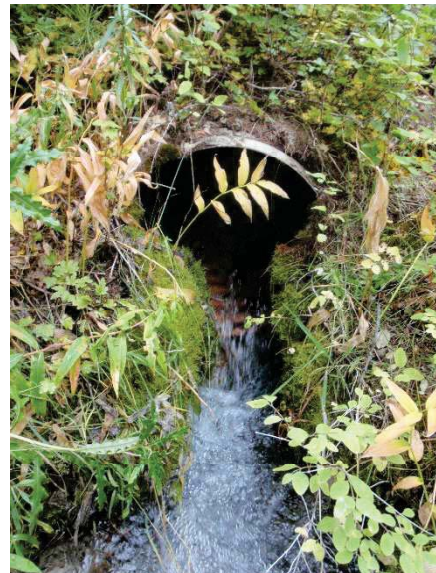
Inlet and outlet of the lower noname creek culvert. It will be replaced with a 102-inch AOP.
