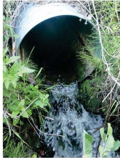
Inlet and outlet of the lower Spring Creek culvert. It will be replaced with a 102-inch AOP.
