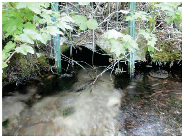
Inlet and outlet of the a second noname creek culvert. It will be replaced with a 48-inch hydraulic culvert.
