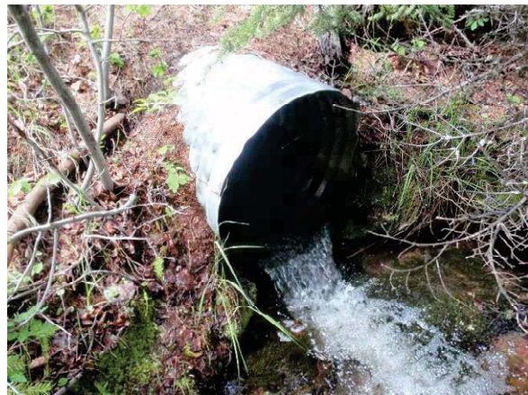
Inlet and outlet of the upper Spring Creek culvert. It will be replaced with a 102-inch AOP.
