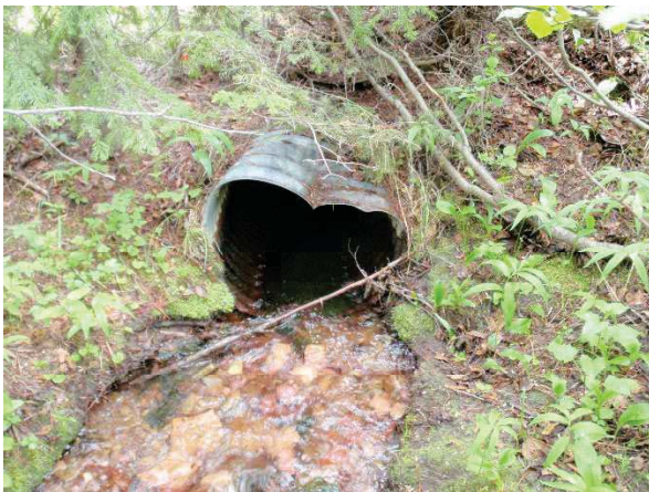
Inlet and outlet of the upper Spring Creek culvert. It will be replaced with a 102-inch AOP.
