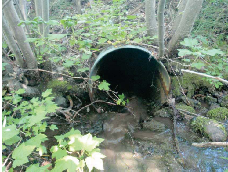
Inlet and outlet of the lower Spring Creek culvert. It will be replaced with a 102-inch AOP.
