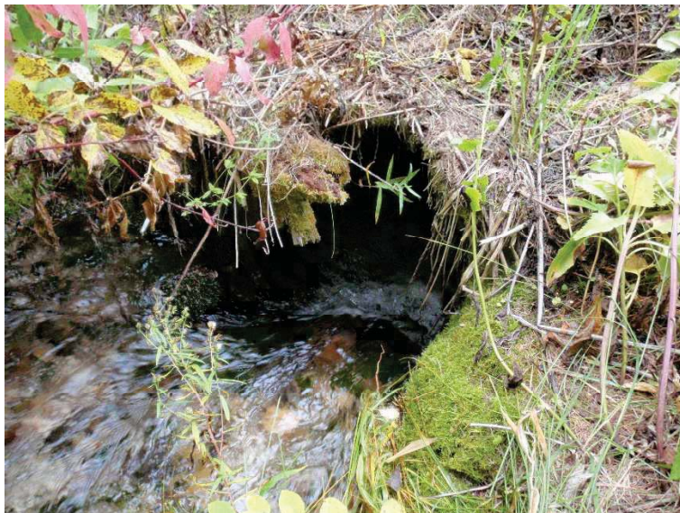
Inlet and outlet of the lower noname creek culvert. It will be replaced with a 102-inch AOP.
