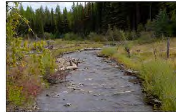
TYPICAL CONSTRUCTED STREAMBED THROUGH A RIFFLE FEATURE
