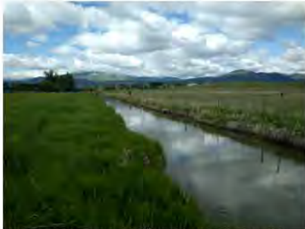
TYPICAL CHANNEL CONDITIONS IN REACH 2, SHOWING STRAIGHTENED, SIMPLIFIED CHANNEL LACKING COMPLEXITY.
