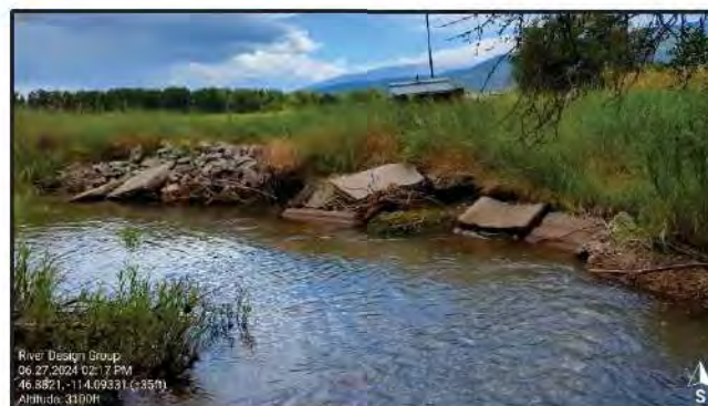
Figure 2-11. Bank stabilization at Station 133+00.
