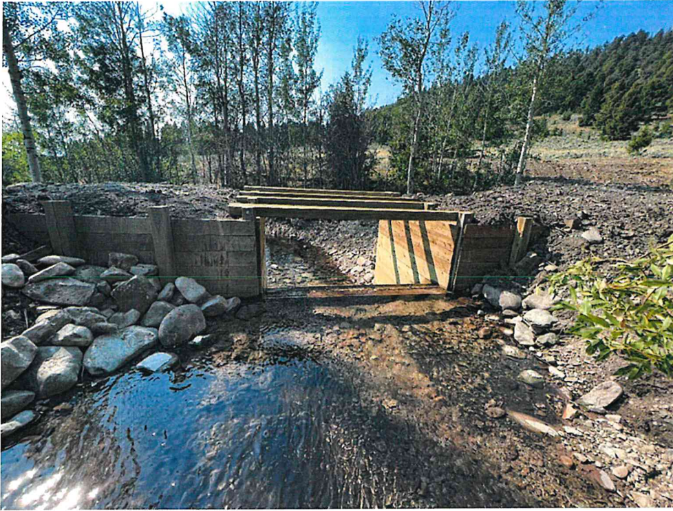
Figure 4. Example of Forest Service constructed wooden plank fish barrier. Photo view is from upstream looking downstream.
