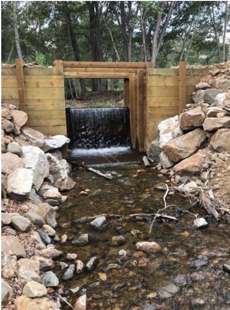
Figure 1. Wooden barrier on Cottonwood Creek in the Beaverhead subbasin. This barrier was installed in 2020 and the stream above the barrier was treated with rotenone for two years. The project was successful, and this population is now considered protected. The barrier on Mono Creek would be a similar design.
