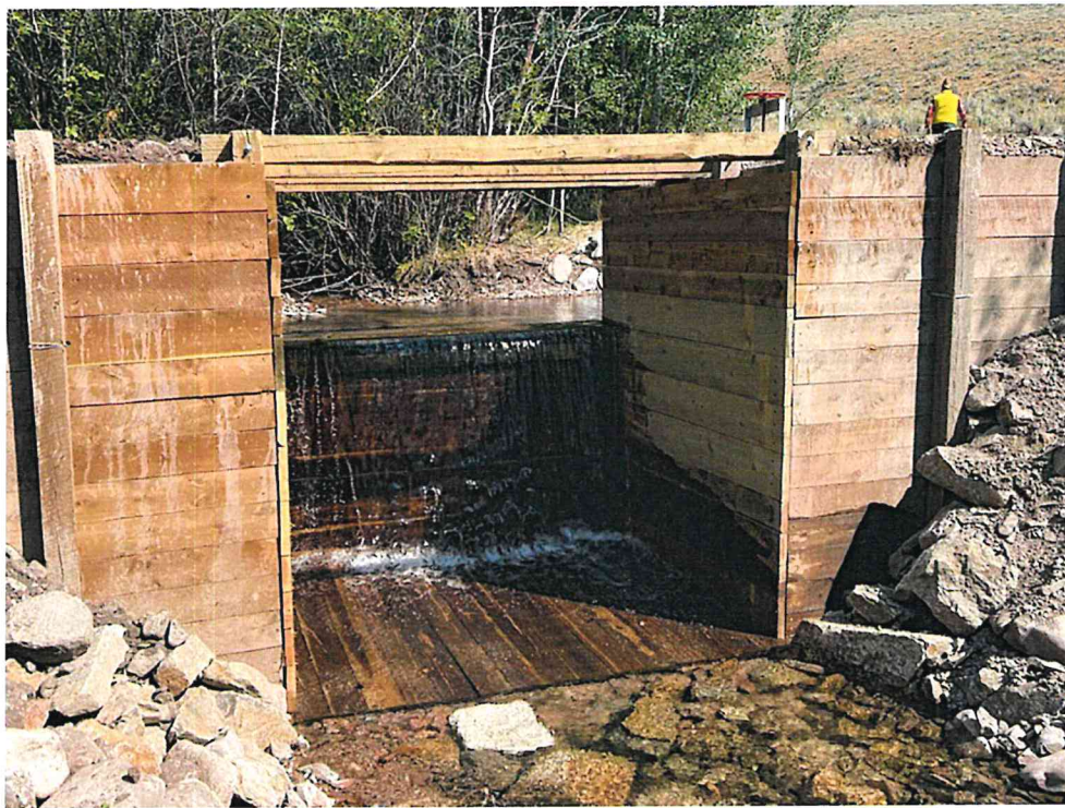
Figure 3. Example of Forest Service constructed wooden plank fish barrier. View from downstream looking upstream.
