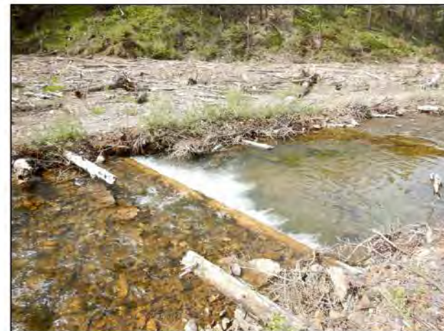
EXAMPLE OF A CONSTRUCTED LOG STEP POOL
