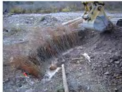
EXAMPLE OF A VEGETATED BRUSH TRENCH INSTALLATION
