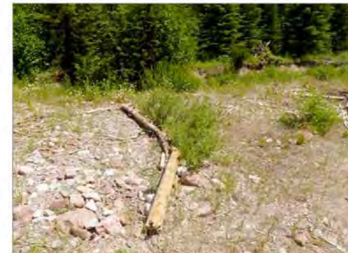
EXAMPLE OF A CONSTRUCTED VEGETATED BRUSH TRENCH
