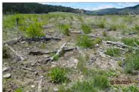
EXAMPLE OF CONSTRUCTED FLOODPLAIN ROUGHNESS
