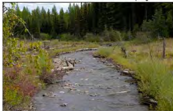
TYPICAL CONSTRUCTED STREAMBED THROUGH A RIFFLE FEATURE
