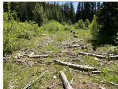
EXAMPLE OF CONSTRUCTED FLOODPLAIN ROUGHNESS
