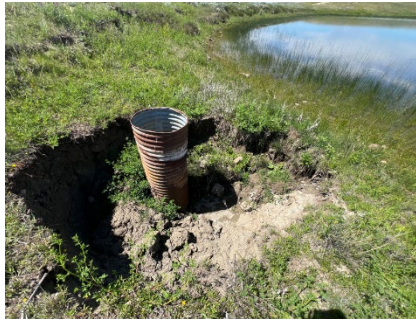
Pictures showing existing condition of trickle tube pipe and active sloughing around structure.
