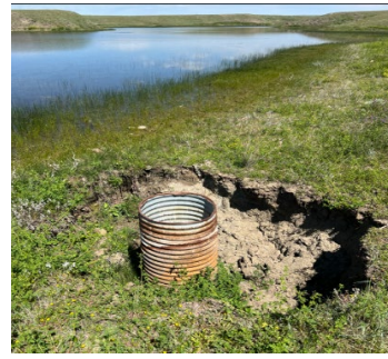
Pictures showing existing condition of trickle tube pipe and active sloughing around structure.
