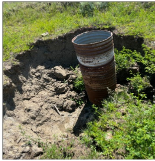
Pictures showing existing condition of trickle tube pipe and active sloughing around structure.
