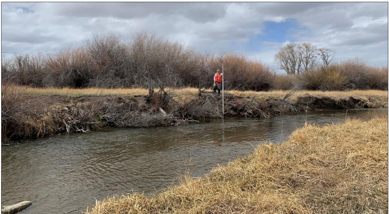
Figure 6. Site PDX4-L (112.68679 °W, 45.17283 °N) is a 145 ft section of degraded stream with a bank height of 4.7 ft. The site recommendation is to slope the streambank back by approximately 14 ft to create an inset floodplain.
