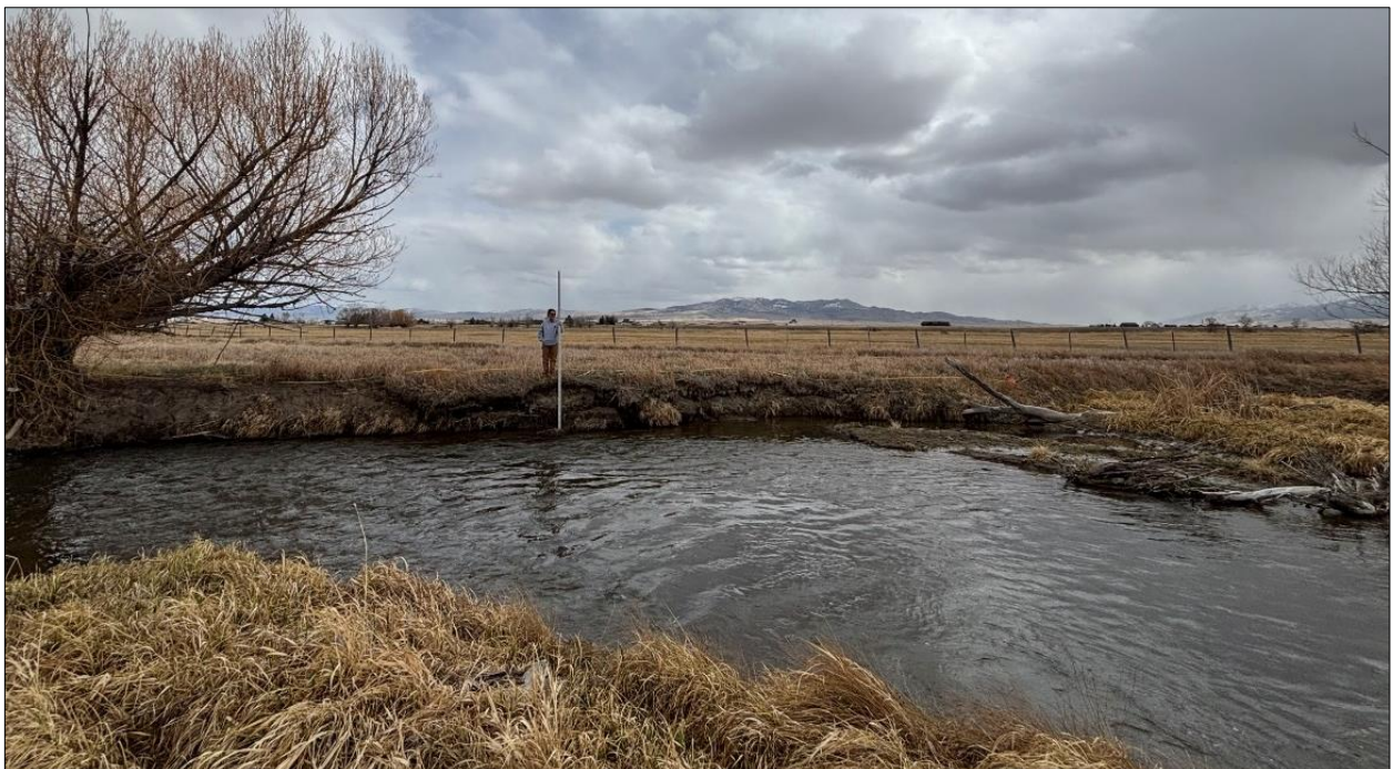
Figure 4. Site PDX2-R (112.68644 °W, 45.17334 °N), a 69 ft long section of degraded bank with a bank height of 3.5 ft at the midpoint. Site recommendation is to slope the bank back by approximately 10.5 ft.
