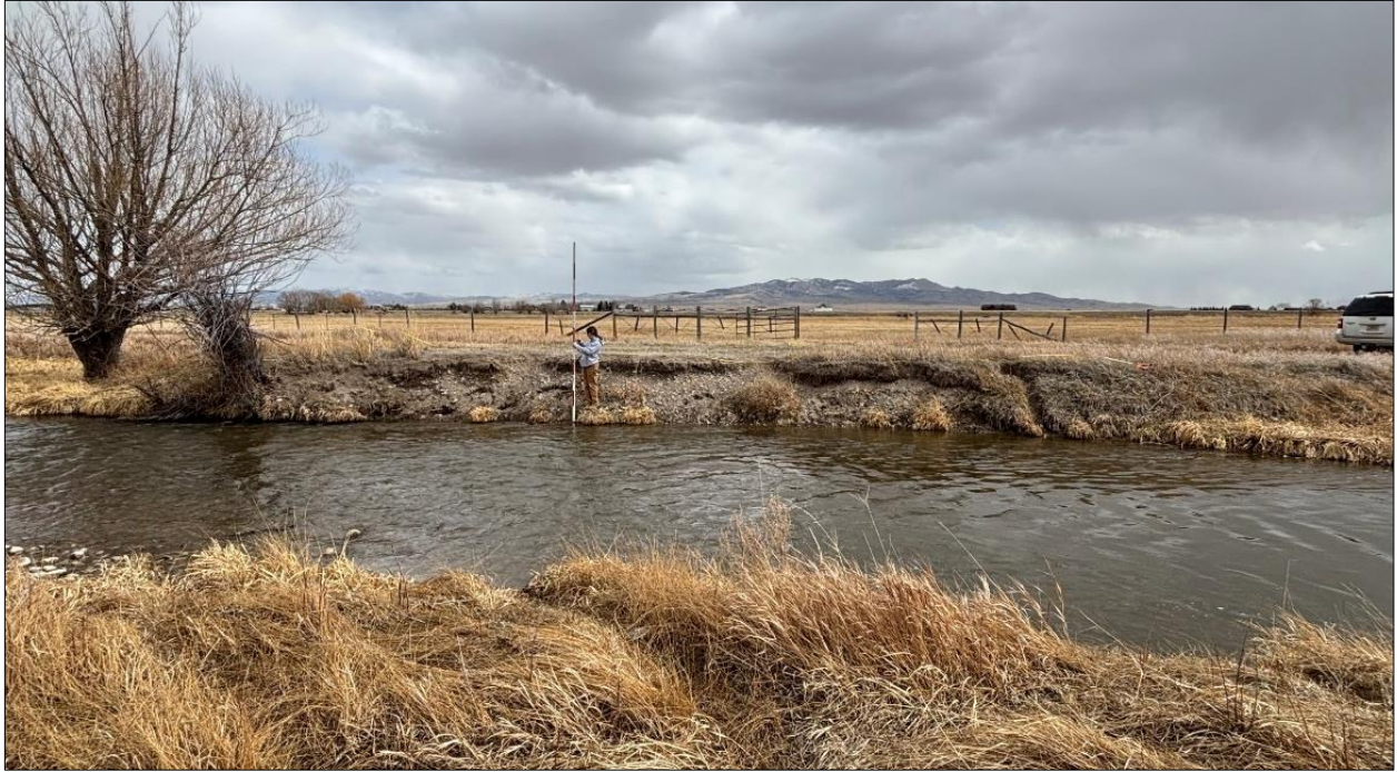
Figure 5. Site PDX3-R (112.68665 °W, 45.17297 °N), a 64.8 ft section of degraded bank with a bank height of 4.3 ft. Site recommendation is to bring back the bank by approximately 12.9 ft.
