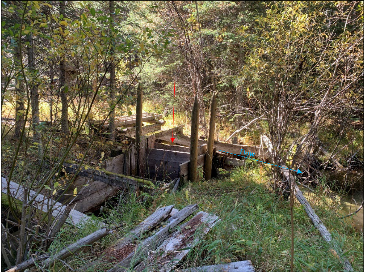
Figure 2. Existing conditions of the old wooden diversion. The red arrow shows the stop logs that lead into the overflow channel (historic channel). These stop logs are no longer in use and create a barrier to fish migrating back into the main channel after being swept into it.
