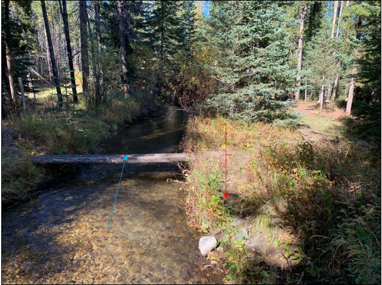
Figure 3. Storm Lake Creek (ditch) immediately downstream of the old diversion structure. This photo illustrates an example of similar low points on the stream bank right (red arrow) that have the potential to overtop and entrain fish at high flows. This bank will be raised with this project.
