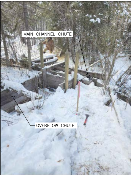
VIEW OF EXISTING TIMBER DIVERSION STRUCTURE LOOKING UPSTREAM AT OVERFLOW CHANNEL CHUTE
