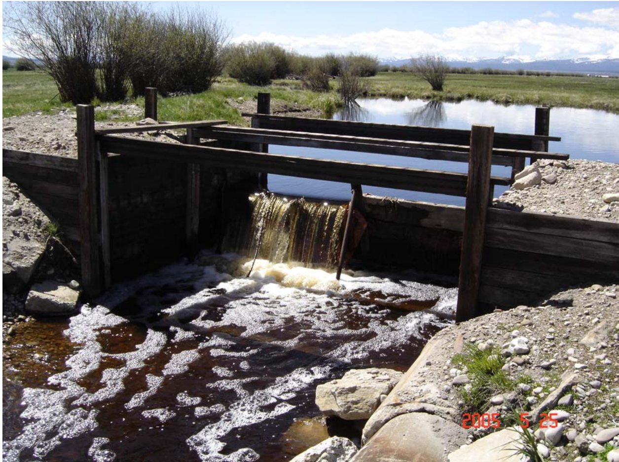
Figure 21. Example of Cross-Channel Diversion Structure in the Project Area That Likely Impedes Grayling Movement But Would Be Remedied Under the Agreement.
