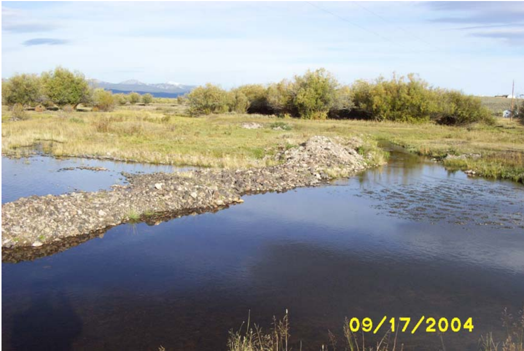
Photo 3G. The current condition of diversion structures on the enrolled land of Landowner “A.” The current diversion is called a “push up” diversion, that is maintained by redistributing (pushing up) streambed gravels with heavy equipment.
