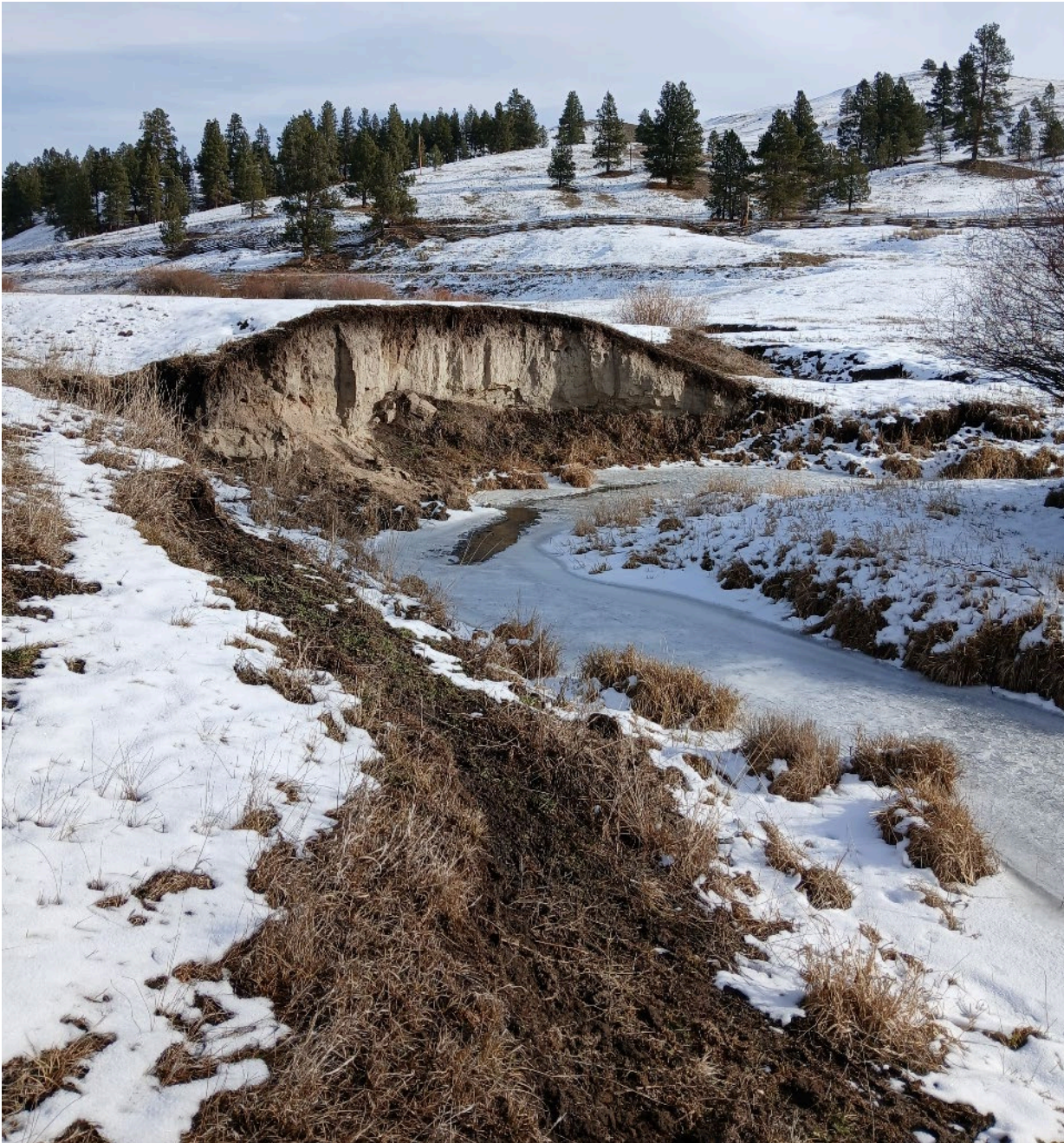
Photo 1, Unit 3: 8-foot tall eroded bank.
