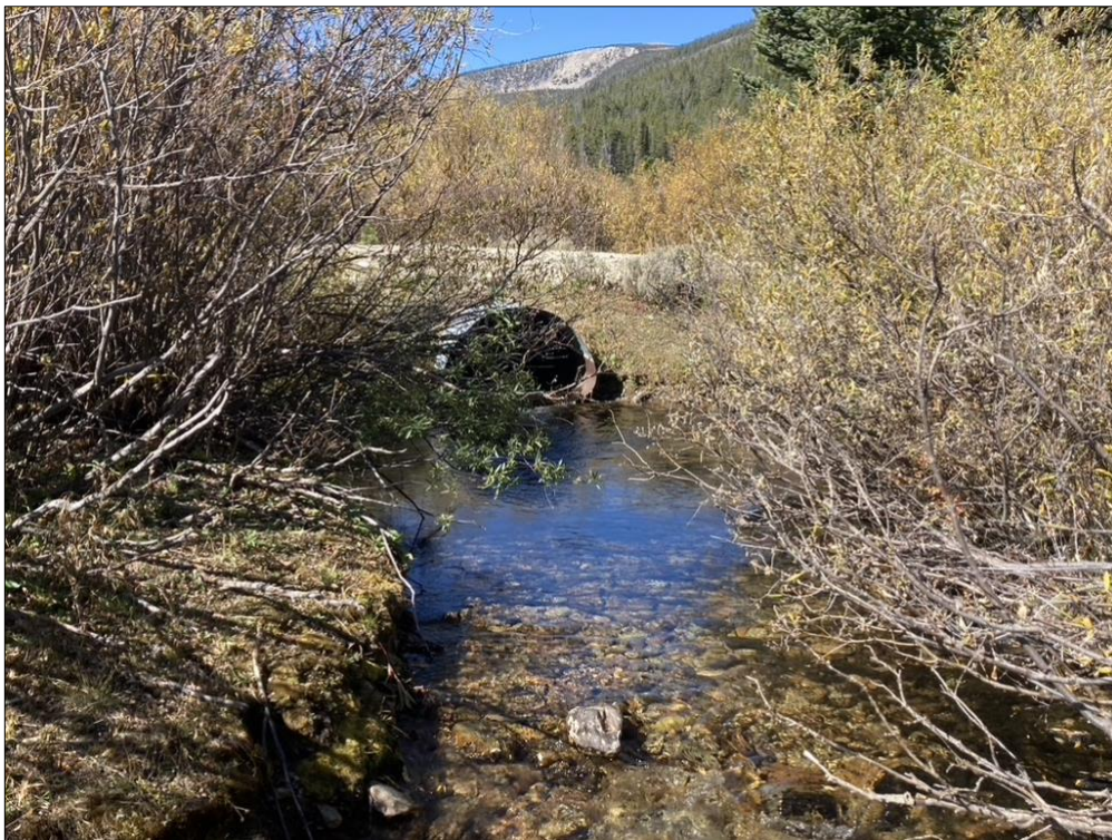
Figure 3. Looking upstream at Darkhorse Creek, 45.17006, -113.52083. One of two (northern) undersized culverts is to be removed and the road obliterated.
