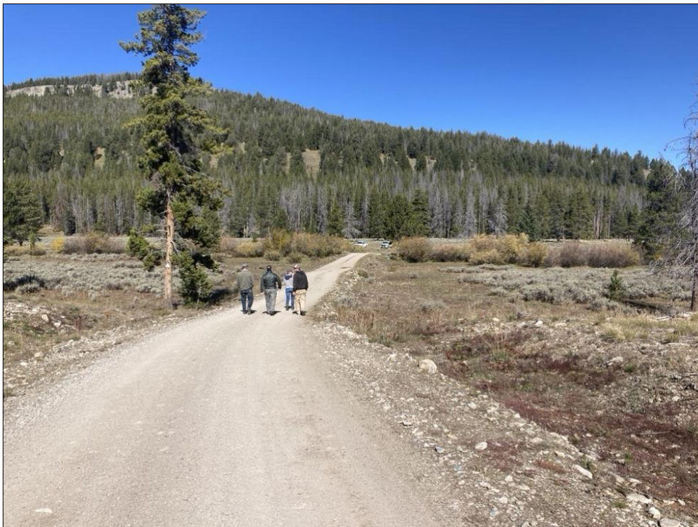
Figure 2. 45.17005, -113.52085, looking north. The current location of USFS Road 381, Skinner Meadows Road, is located on an alluvial fan, causing ponding and excess sediment to the Big Hole River. The road is an important corridor leading to several public fishing opportunities, including the upper Big Hole River, Darkhorse Creek, Van Houten Lake, Reservoir Lake, Bloody Dick Creek, and Selway Creek.
