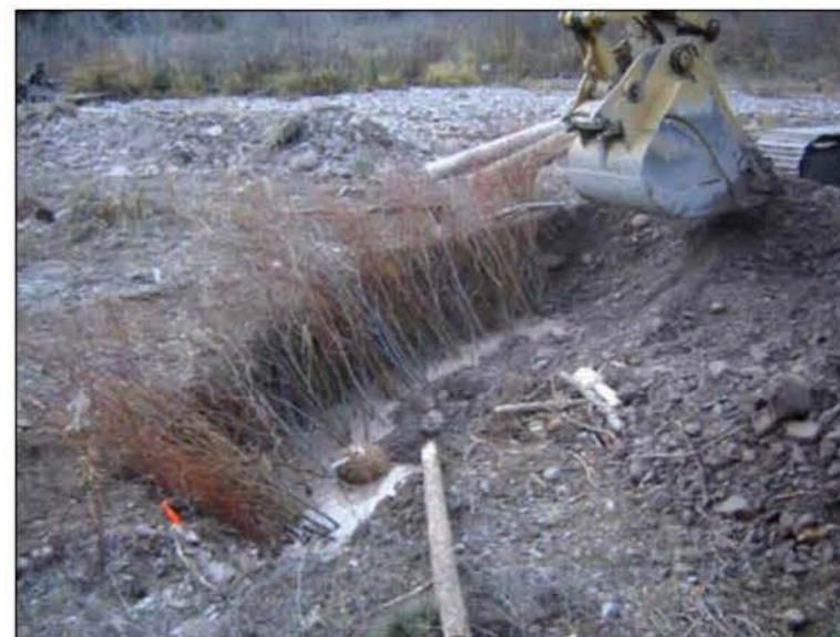
EXAMPLE OF A VEGETATED BRUSH TRENCH INSTALLATION
