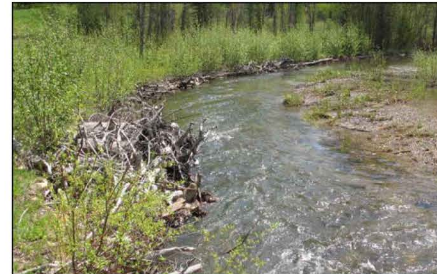
TYPICAL CONSTRUCTED STREAMBED THROUGH A RIFFLE FEATURE
