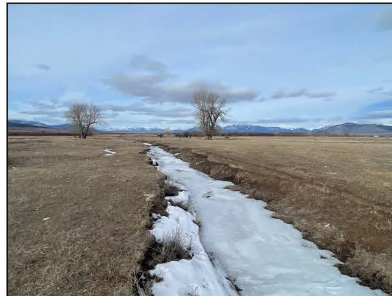
A MAJORITY OF REACH 2 WAS HISTORICALLY STRAIGHTENED AND CHANNELIZED TO ACCOMMODATE AGRICULTURAL LAND USES. THIS RESULTED IN CHANNEL INCISION AND LOSS OF FLOODPLAIN CONNECTION. HABITAT IS EXTREMELY SIMPLIFIED AND DOMINATED BY RIFFLE HABITAT UNITS WITH LIMITED POOL DEVELOPMENT.
