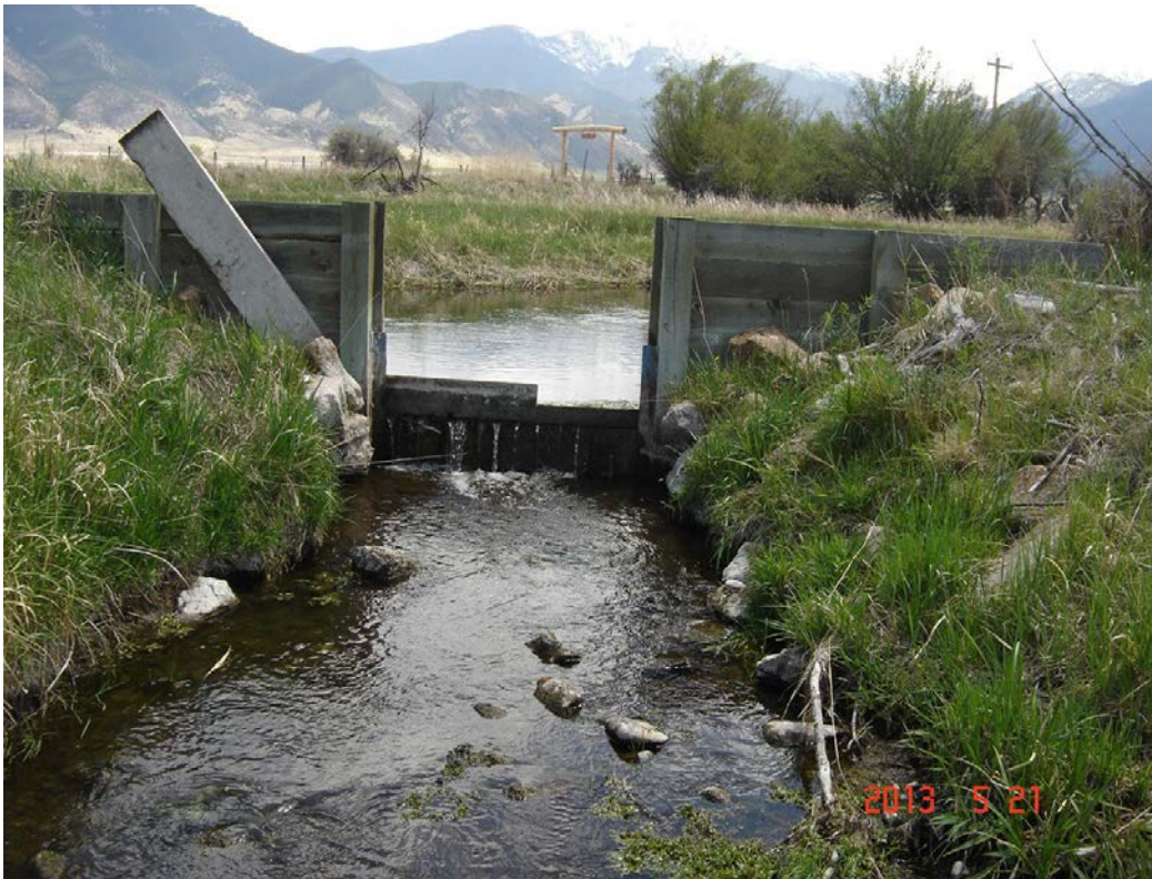
Figure 8. View looking upstream at the spawning channel diversion with check-boards (stop logs) installed. At certain times, low flow conditions occur in the spawning channel when water is being diverted down the irrigation ditch.
