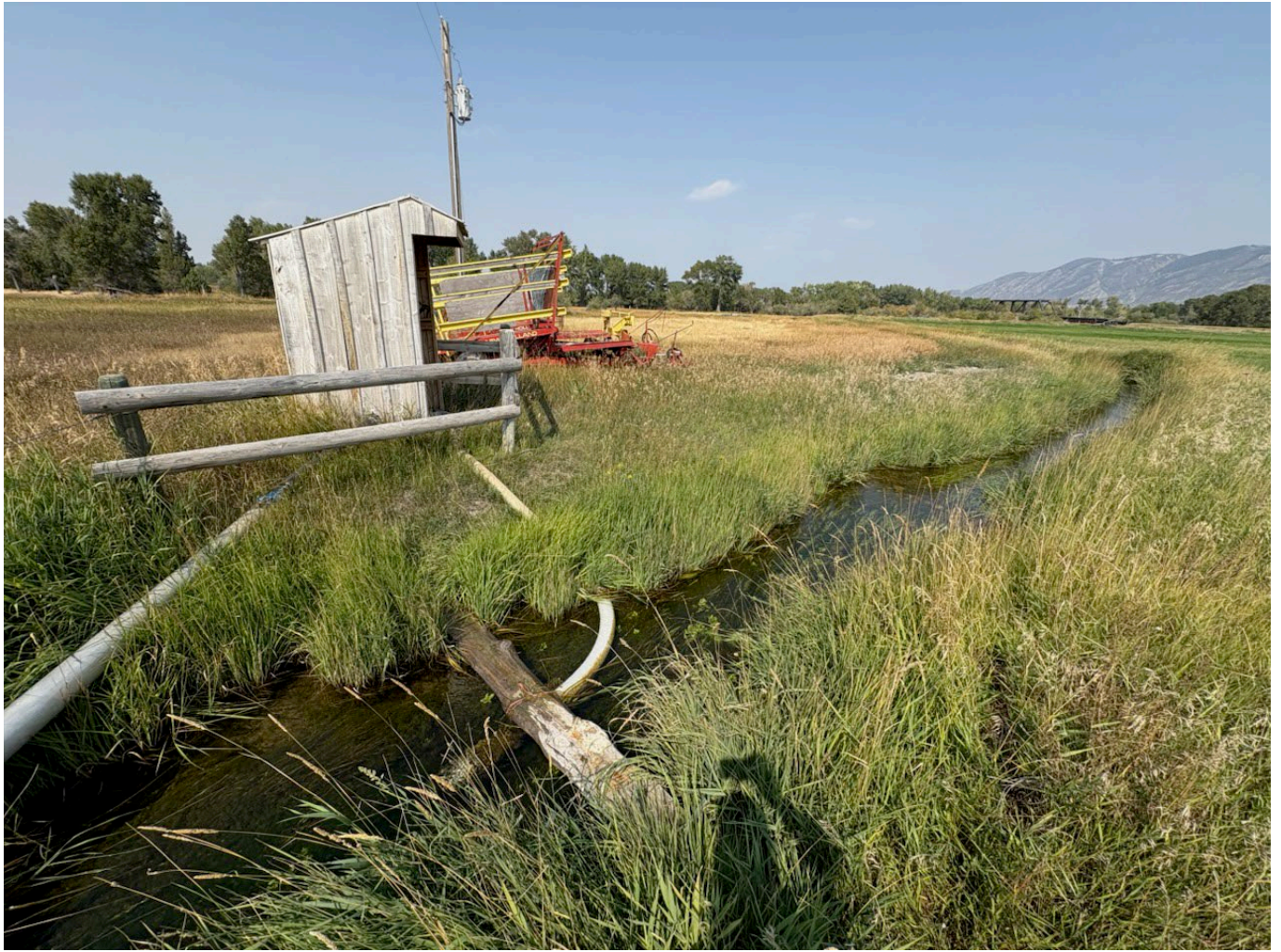
Figure 5. Photograph of the existing Laughery pump site on the Parsons Ditch. The ditch flows from left to right in the image. The Parsons Railroad Bridge can be seen along the tree line.
