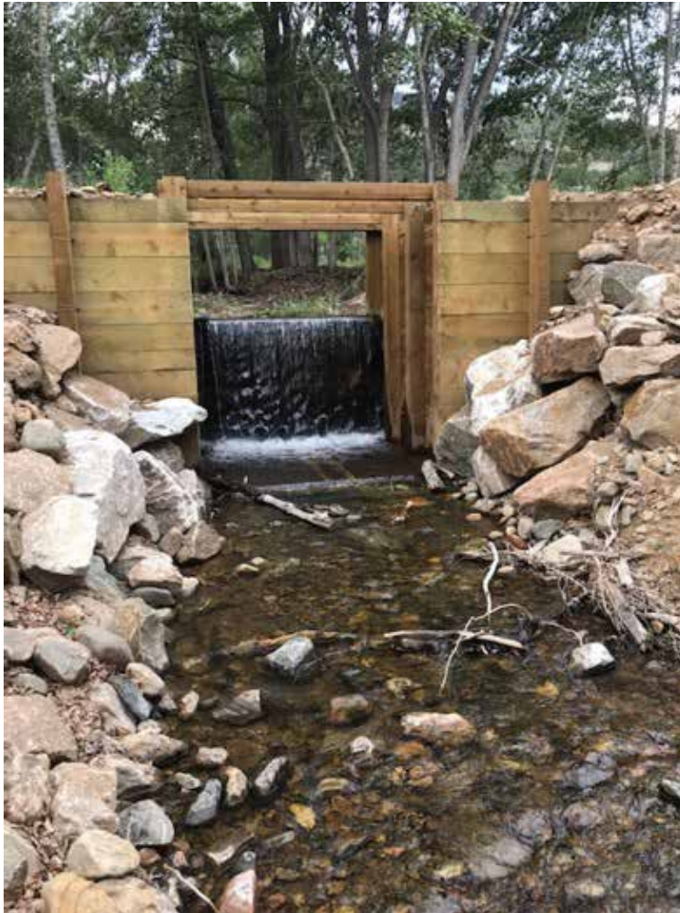
Figure A. Wooden barrier on Cottonwood Creek in the Beaverhead River subbasin. This barrier was installed in 2020 and the stream above the barrier was treated with rotenone for two years. The project was successful, and this population is now considered protected. The barrier on Red Rock Creek would be a similar design.
