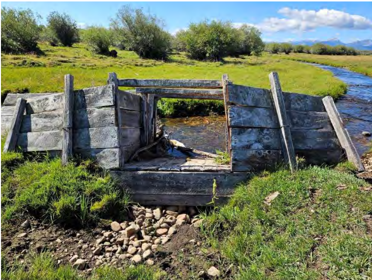
Pin and plank that was once in Rock Creek to divert flows into the ditch, is now on the bank.
