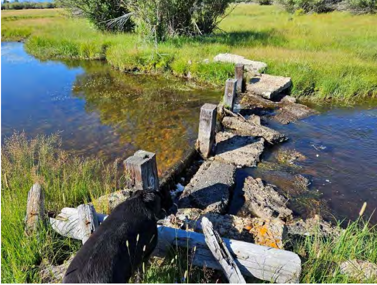
Old pin and plank across Rock Creek blocking fish passage.
