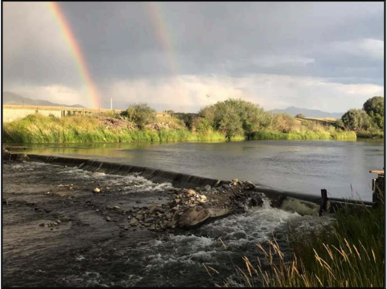
Figure 4: Existing Jersey Barrier on Side Channel 45.62274 N, 112.31086 W
