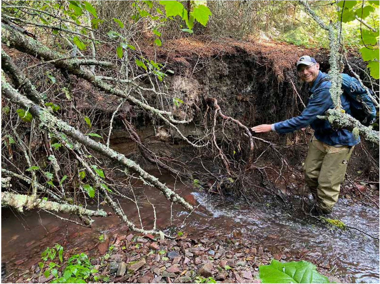
Figure 5: Another example of an actively eroding bank that will be treated.
