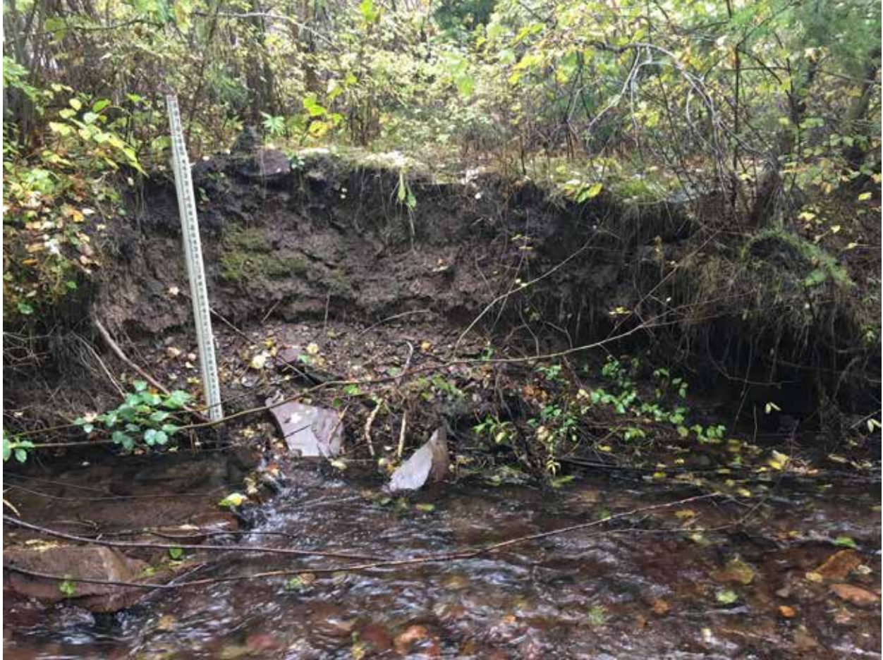
Figure 4: Bank erosion is severe at several sections of the creek. They will be treated with vegetated wood matrix and large wood structures creating inset floodplains.
