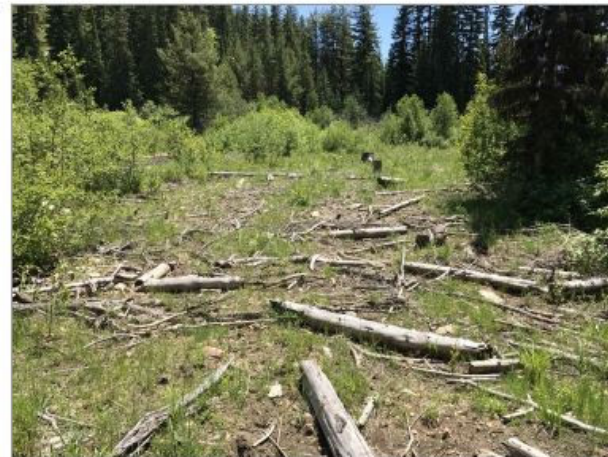
EXAMPLE OF CONSTRUCTED FLOODPLAIN ROUGHNESS
