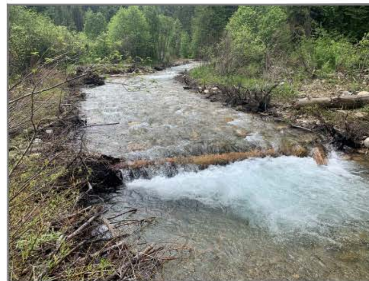
TYPICAL CONSTRUCTED STREAMBED THROUGH A RIFFLE FEATURE
