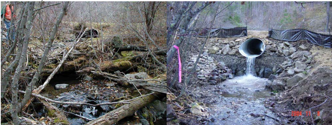
Figure 11. Photograph of old culvert and new culvert barrier on Middle Fork Little Belt Creek, 2004.
