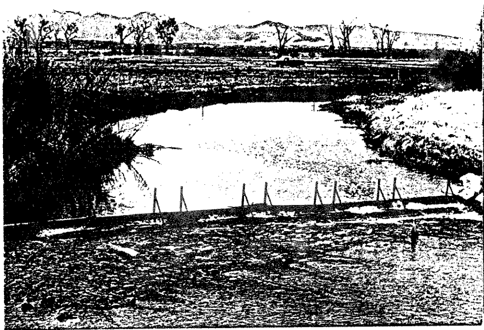
Figure 1. Portable steel plate alternative irrigation diversion structure in place on the Beaverhead River. Beaverhead County.
