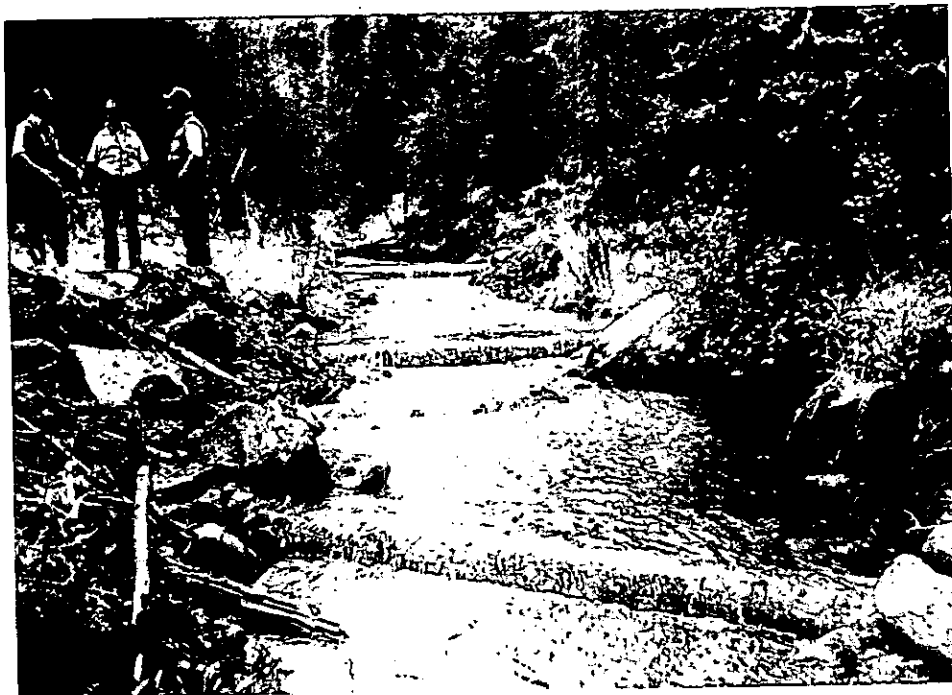
Figure 10. View of the deteriorating log bridge on Trapper Creek prior to its removal (top) and following its removal and placement of log sills to hold spawning gravels (bottom).
