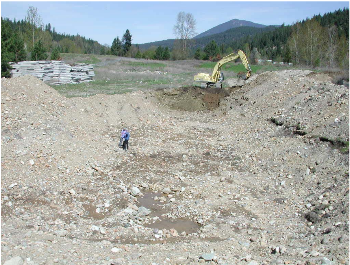
Figure 6. Photographs of the excavation of Troy Fish Pond and removal of fill material. Weeded area shows level of fill.
