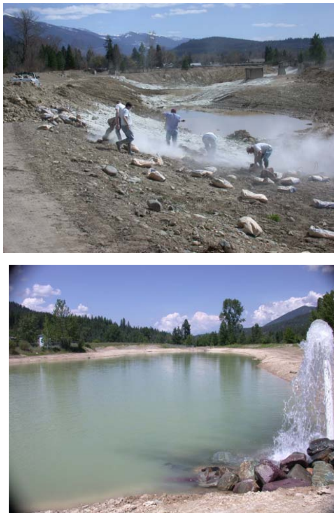
Figure 7. Photographs of the Troy fishing pond during bentonite application and shortly after construction during the 2002 summer.
