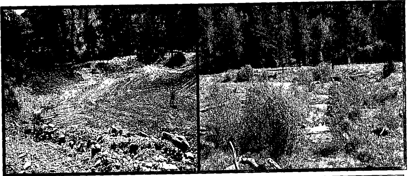
Channel reconstruction: These photos show a bulldozed channel (left) before reconstruction and the newly reconstructed channel (right). The new channel included sod transplants and instream wood for bank stability and habitat.
