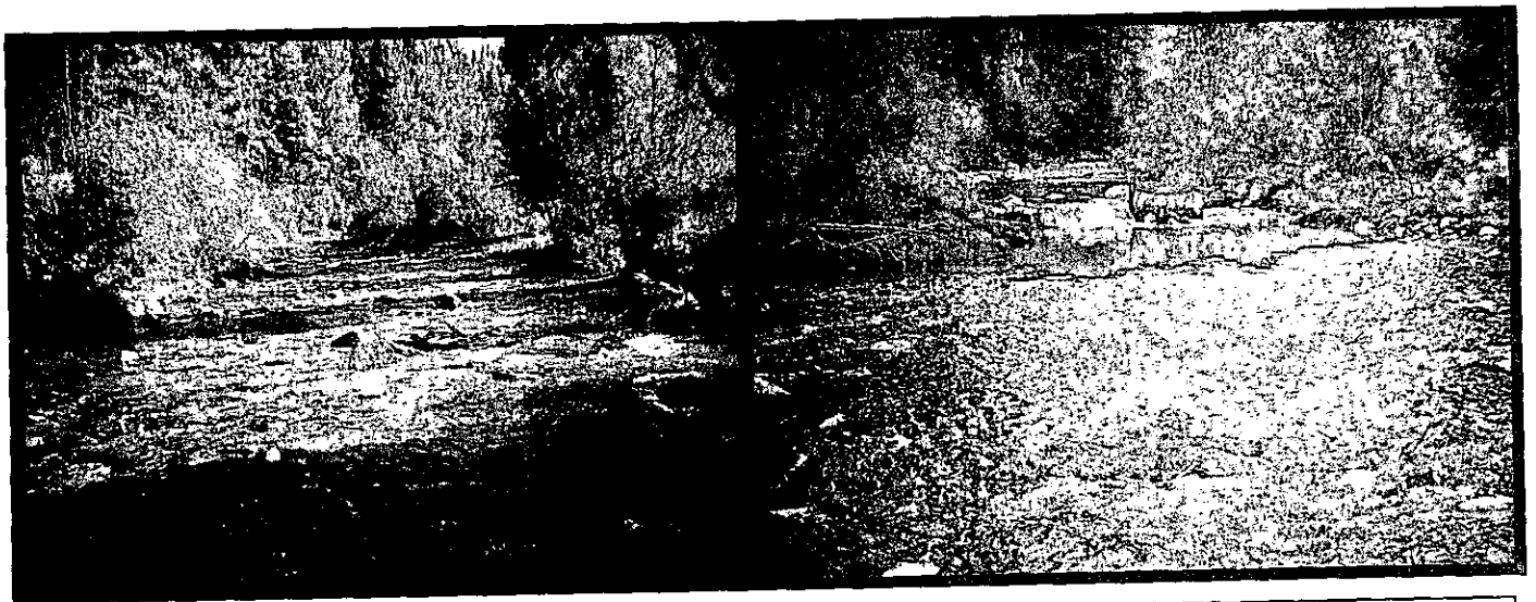
Instream habitat restoration: These photos show a stream of moderate gradient before (left) and after instream habitat restoration (right), using all native materials (wood and on-site rock). Before instream habitat restoration, this stream had all large wood removed from the channel, leading to the loss of pools and loss of habitat complexity.
