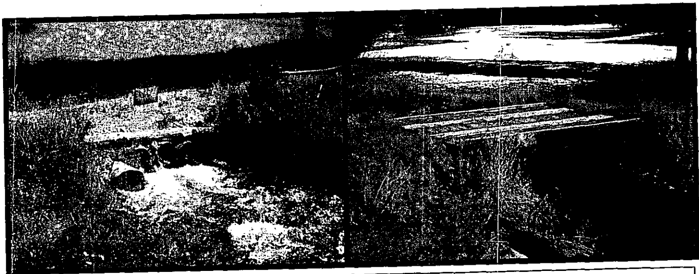
These photos show a culvert replacement project. The culverts were high velocity barriers to small fish. Bridges allow unimpeded upstream fish passage, plus allows upstream movement of other species like amphibians, which rely on natural stream bottoms.
