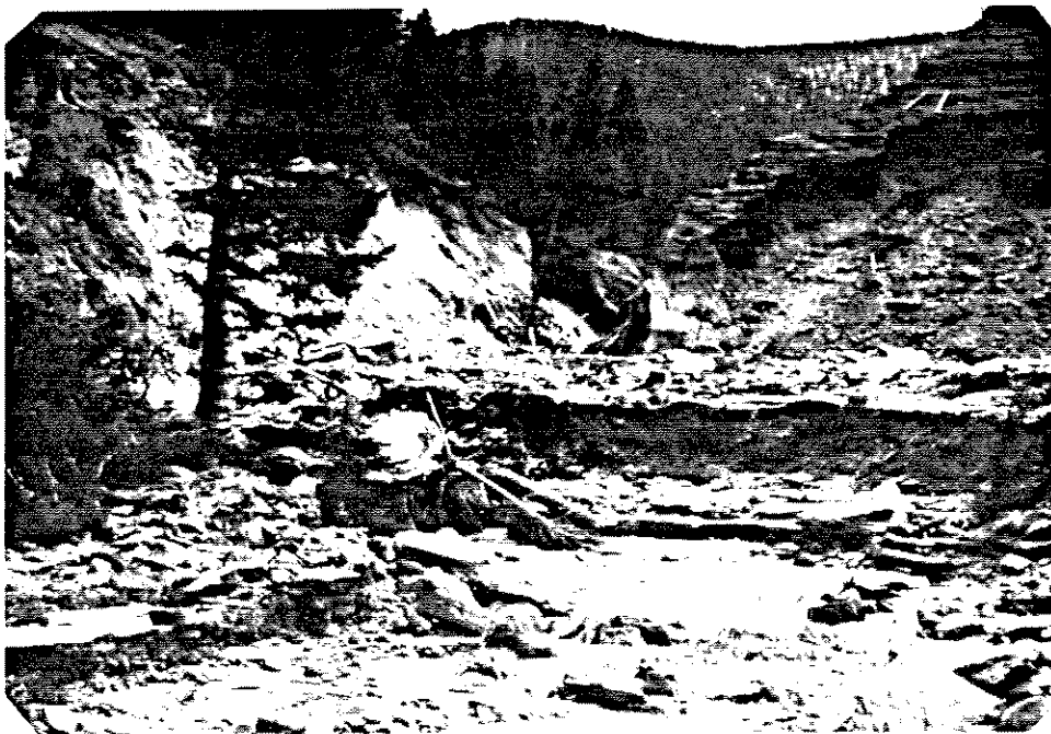
Photo 4. Breach in Mike Horse Dam, looking at dam from downstream. West side of breach is on the right. June 24, 1975.
