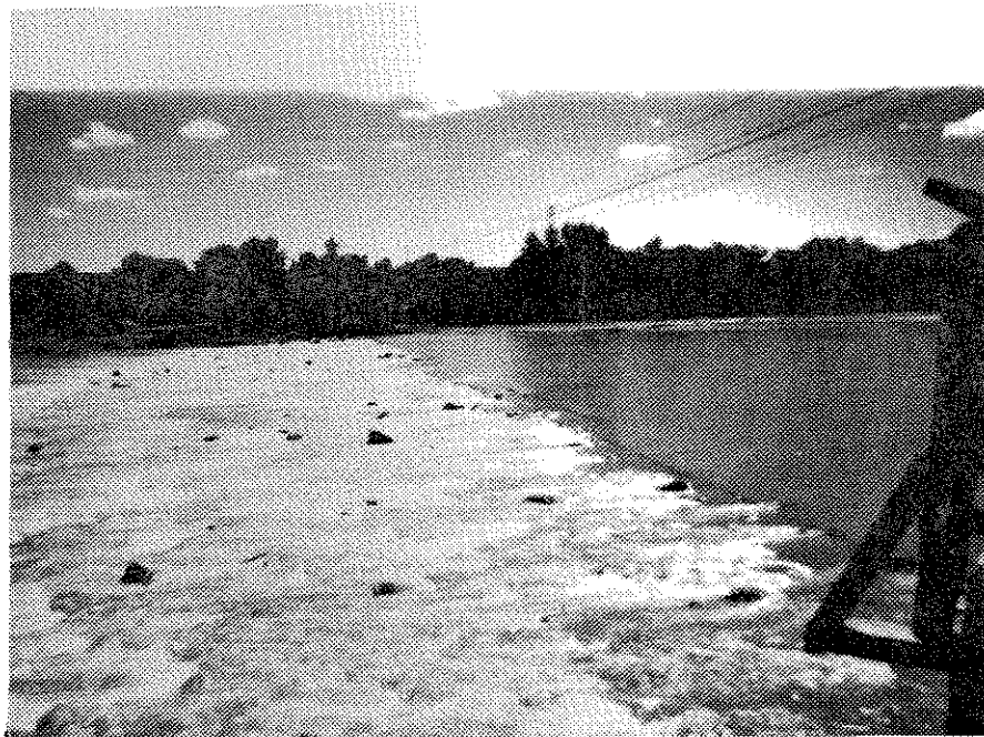
Figure 3. Intake diversion is a submerged, wooden-framed structure covered with large boulders.
