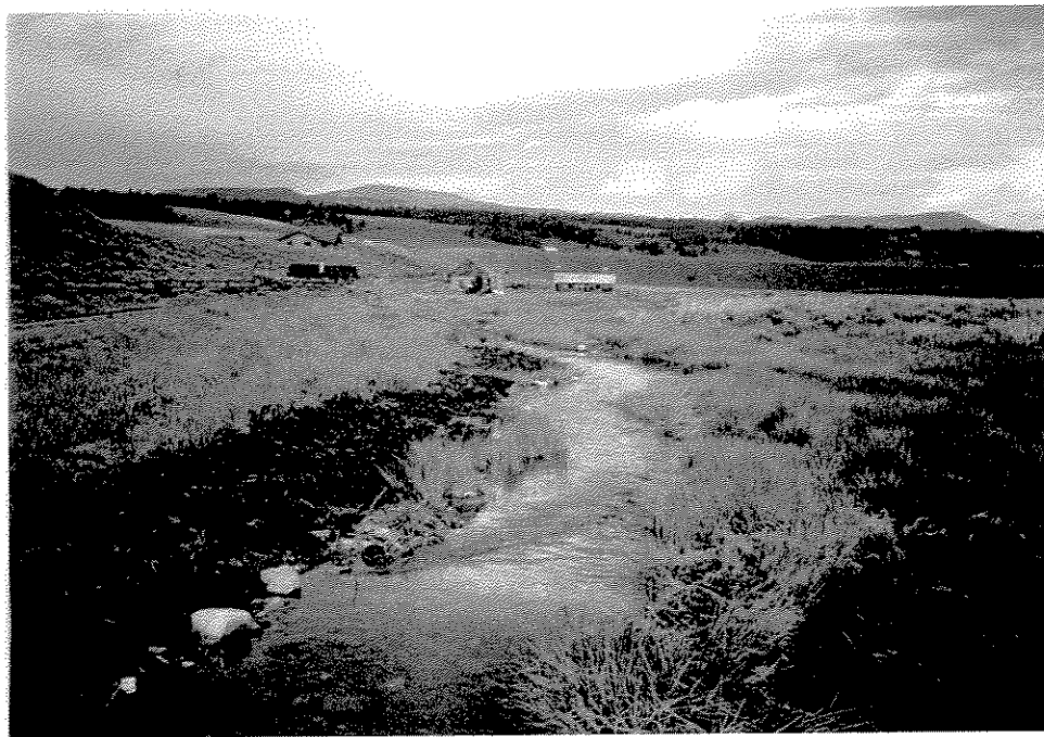
Photo illustration 2. Madison Spring Creek, which enter the Madison River near the Wade lake cut-off, before and immediately after restoration. The stream has been narrowed and deepened to increase current velocity, facilitate sediment transport, and create cover for fish.
