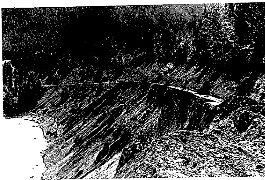
Figure 8. Destruction of U.S. Highway 2 along Middle Fork Flathead River on Flathead National Forest (Photo courtesy U.S. Forest Service).
