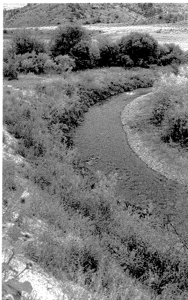
Photo illustration 1. Deep Creek (east of Townsend) during and after treatment of a steep eroding bank. Banks were back sloped and stabilized with juniper bundles cabled into the slope. Willows will eventually provide more permanent bank stability.
