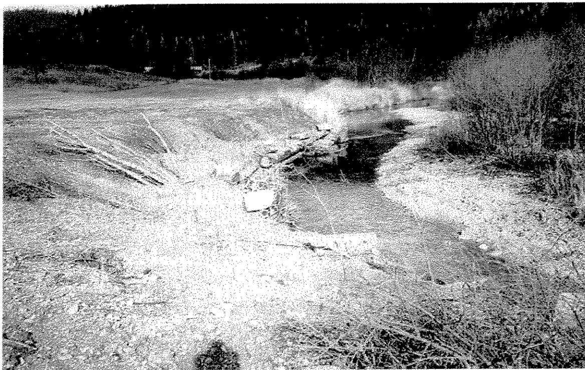
Photo illustration 2. Elk Creek (near Heron) before and immediately after restoration. The channel was reshaped and banks were stabilized using root wads, boulders, and log footers. The new channel is deeper and more diverse — providing better fish habitat.
