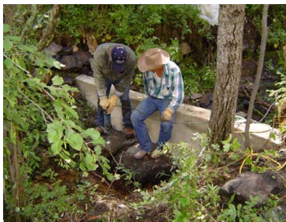
Construction of Crawford Creek fish barrier.
