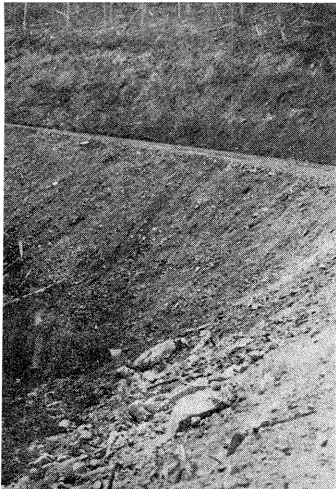
Photo 24. Steep, unvegetated, and unstable cut and fill slopes along Pickfoot Creek.
