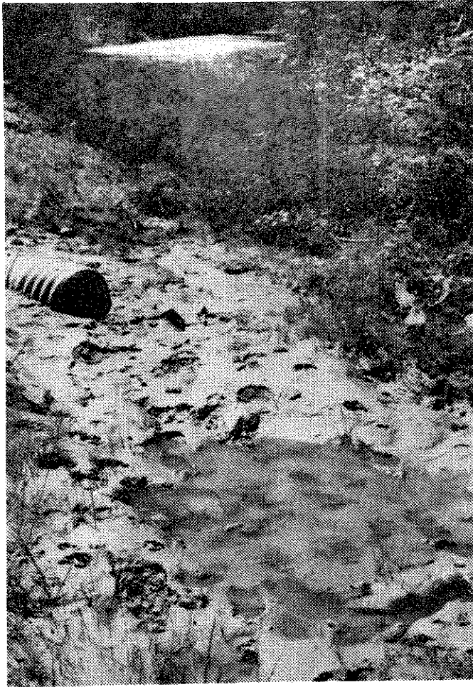
Photo 16. Sediment collecting below a culvert in the East Fork of Lolo Creek.
