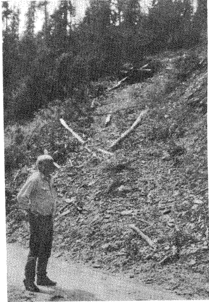
Photo 13. A well designed skid trail in the Freeland Creek drainage. The skid trail has been water-barred and debris piled to prevent runoff from being channeled to the road below.
