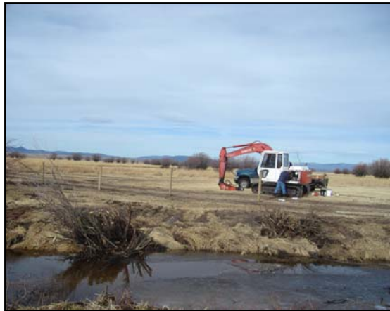
Installing riparian fence along Rock Creek
