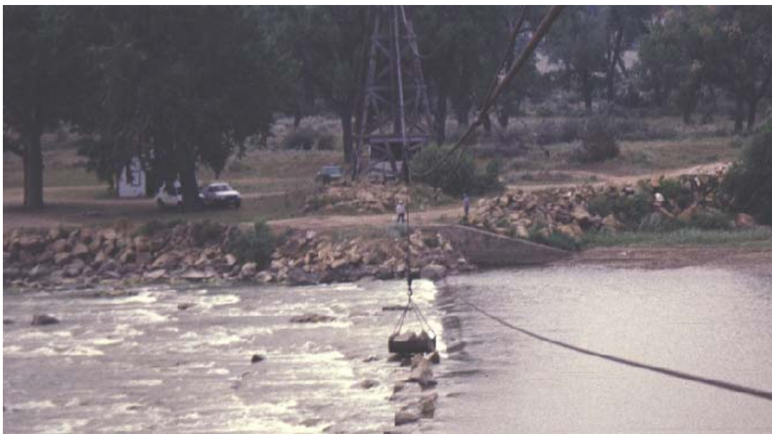
Figure 2 – Intake Diversion Dam Replacing Crest Rock
