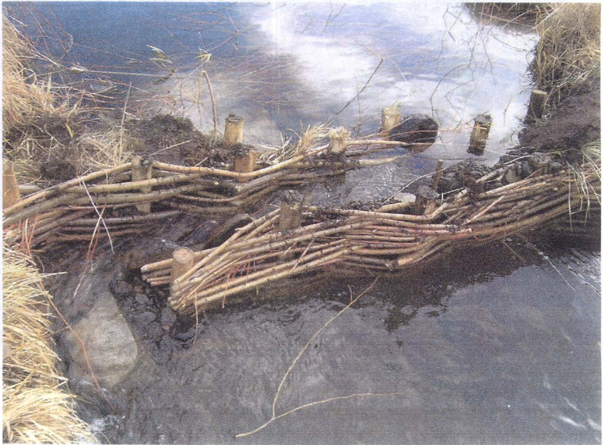
Figure 4. Gazelle Creek willow wicker weir structure. Note the fish passage ramp design.
