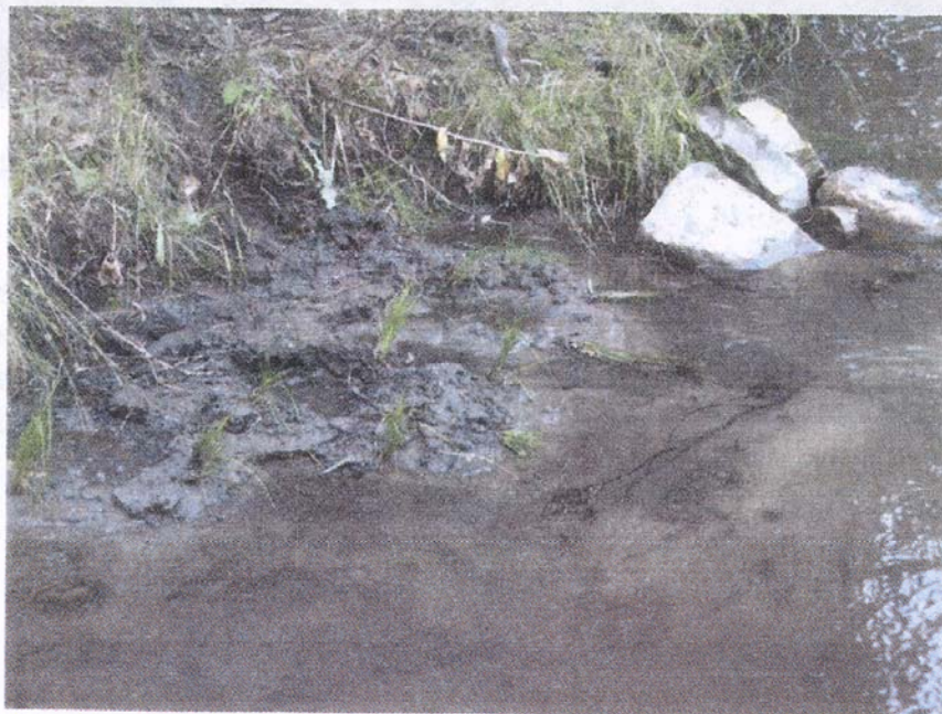
Figure 4. Sedge plugs in fine sediment deposited behind a baffle.
