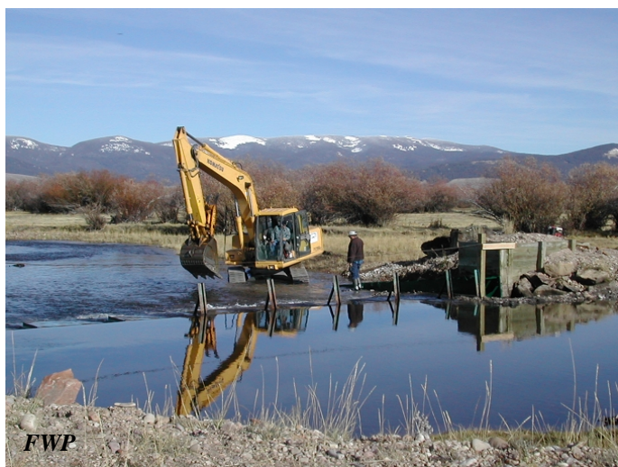
Installing a fish ladder to improve fish passage on the Big Hole River
